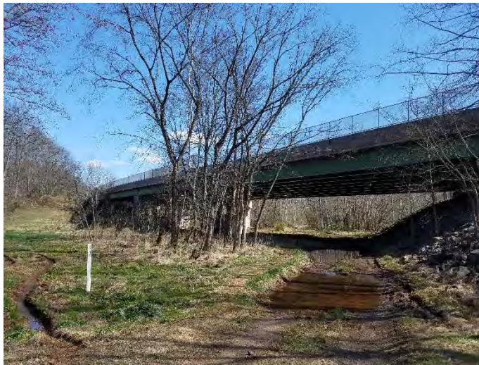
Figure 4-3 - Algonkian Parkway Bridge Traveling over Sugarland Run
