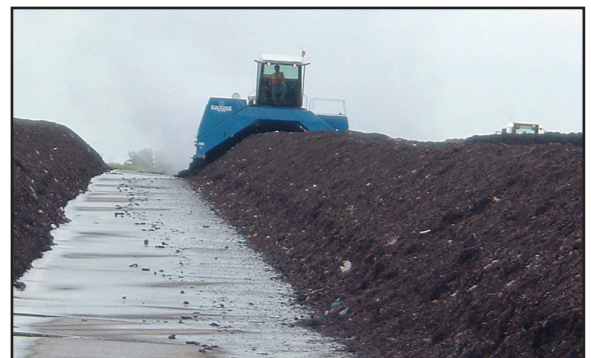
Windrow turner in operation at the Montgomery County Composting Facility.
